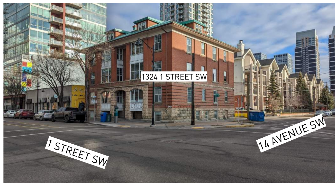
1 EXISTING SITE PHOTO FACING NORTHEAST N/A
