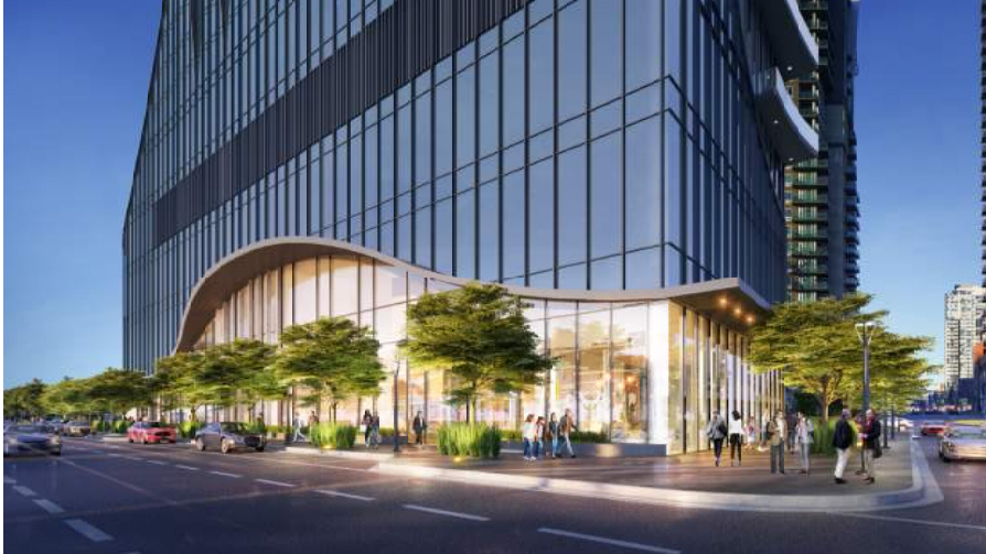
STREET VIEW - NORTH-EAST
