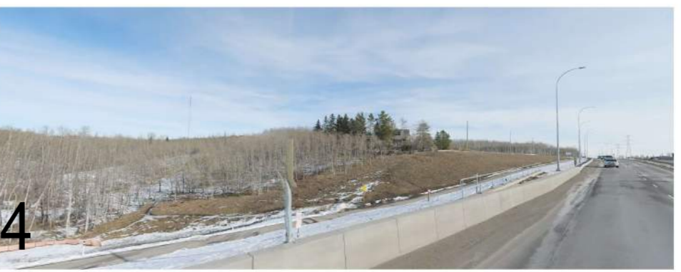
VIEW 04 FROM BOW TRL. SW LOOKING NE
