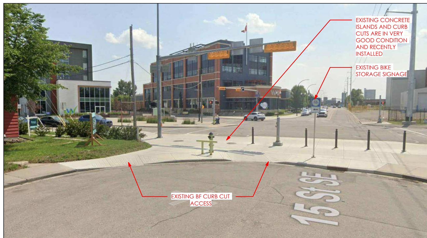
EXISTING SOUTHWEST CORNER VIEW OF CONCRETE CURB, RAMP AND SIDEWALK
