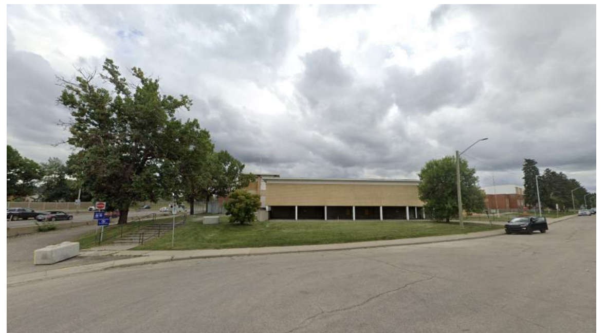
B - SITE PHOTOGRAPH - NORTH EAST CORNER
