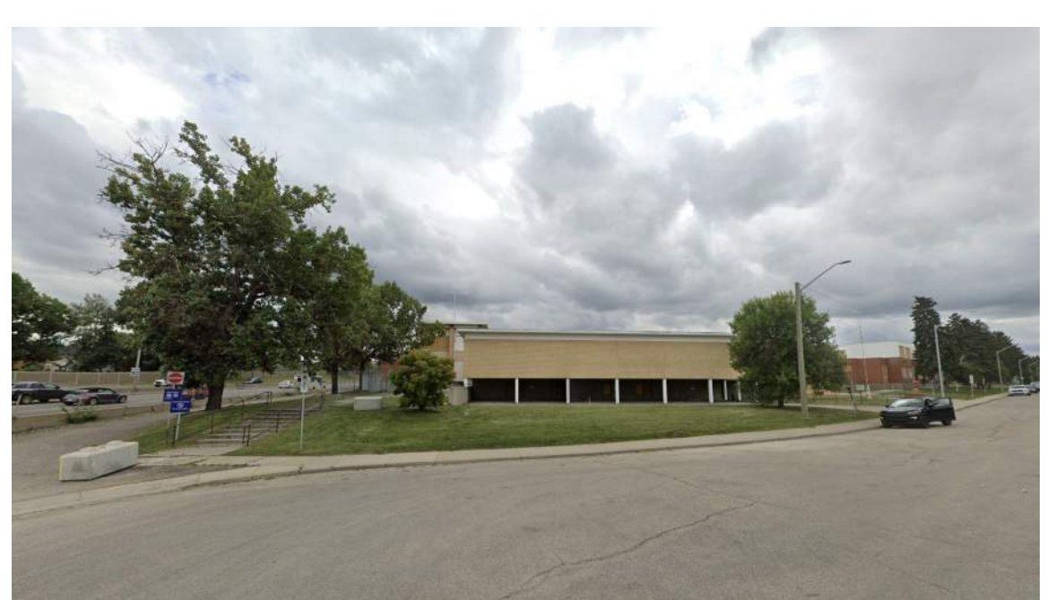
B - SITE PHOTOGRAPH - NORTH EAST CORNER
