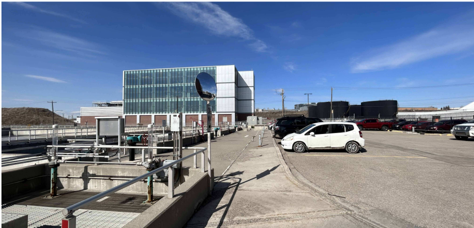
4 BONNYBROOK SITE SOUTH PARKING - LOOKING WEST
