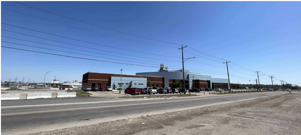
1 BONNYBROOK SITE WEST FROM 15TH STREET SE
