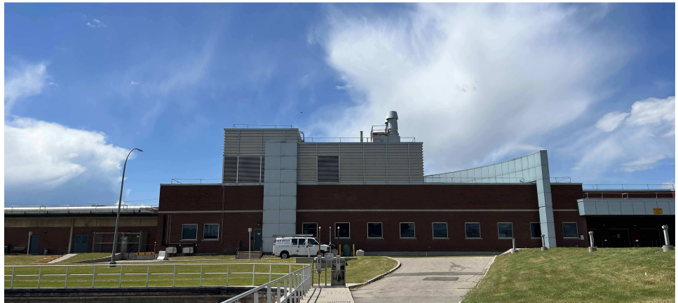
2 BONNYBROOK SITE EAST FROM SECURED AREA
