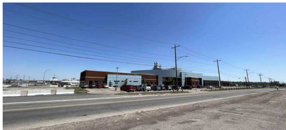
1 BONNYBROOK SITE WEST FROM 15TH STREET SE
