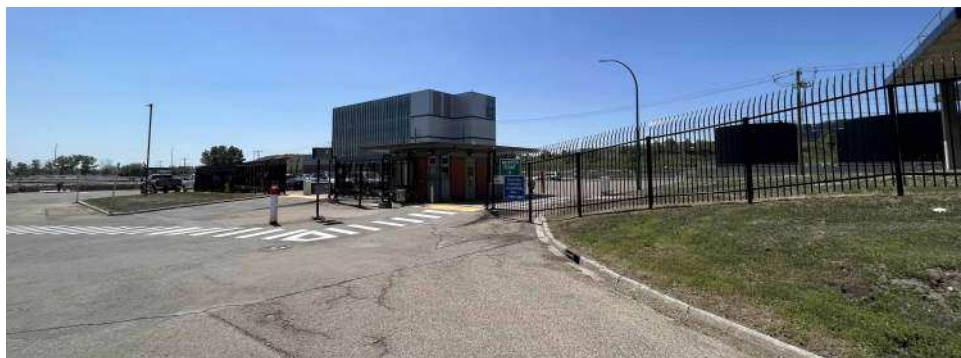
5 BONNYBROOK SITE GATEHOUSE - LOOKING WEST
