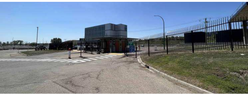
5 BONNYBROOK SITE GATEHOUSE - LOOKING WEST
