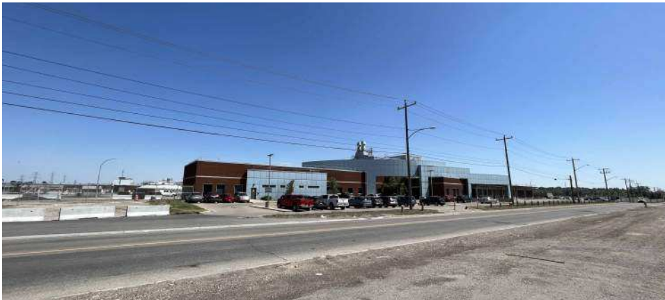
1 BONNYBROOK SITE WEST FROM 15TH STREET SE
