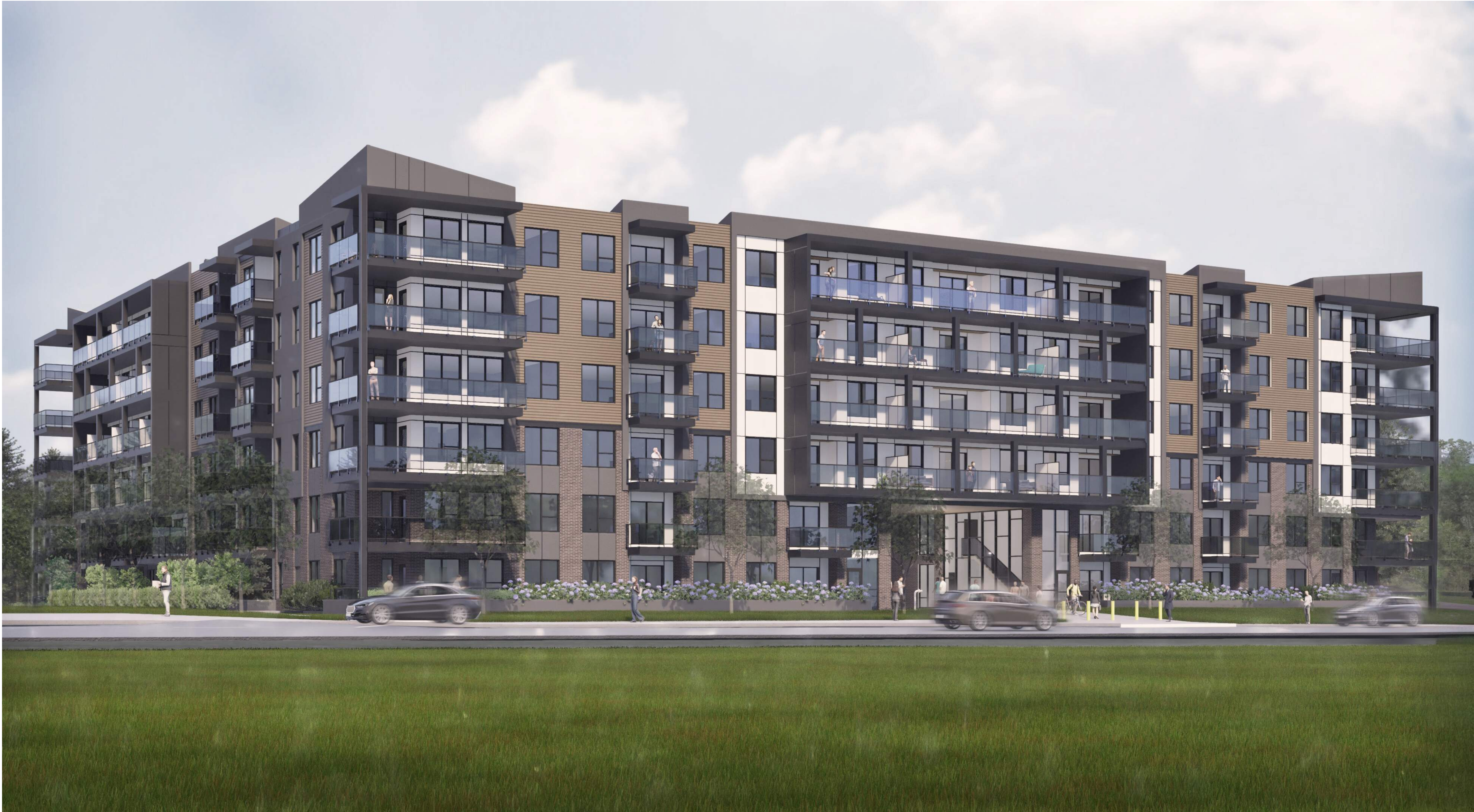
SW CORNER AT 17TH AVENUE
