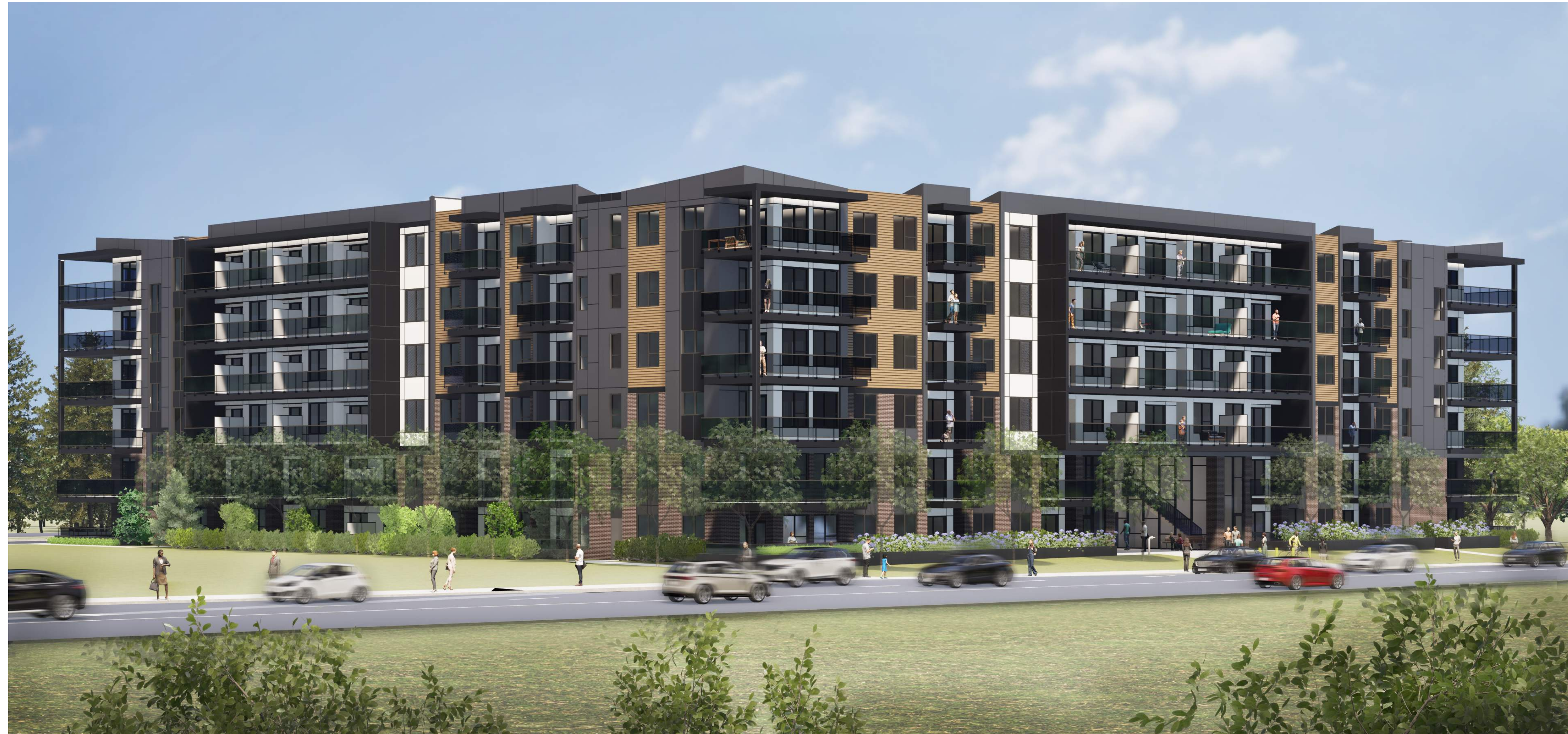
SOUTH/WEST CORNER OF DEVELOPMENT
