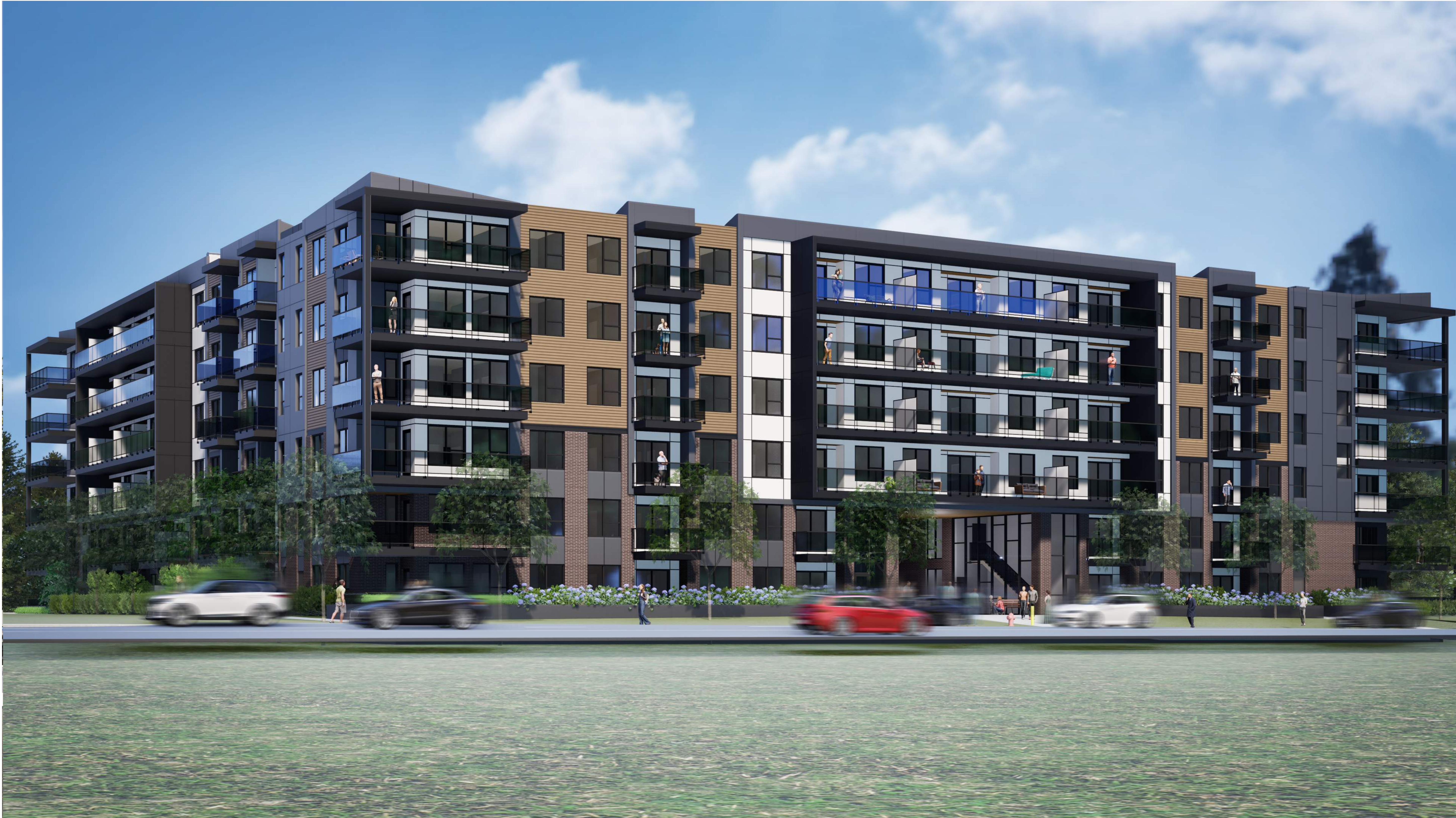
SW CORNER AT 17TH AVENUE
