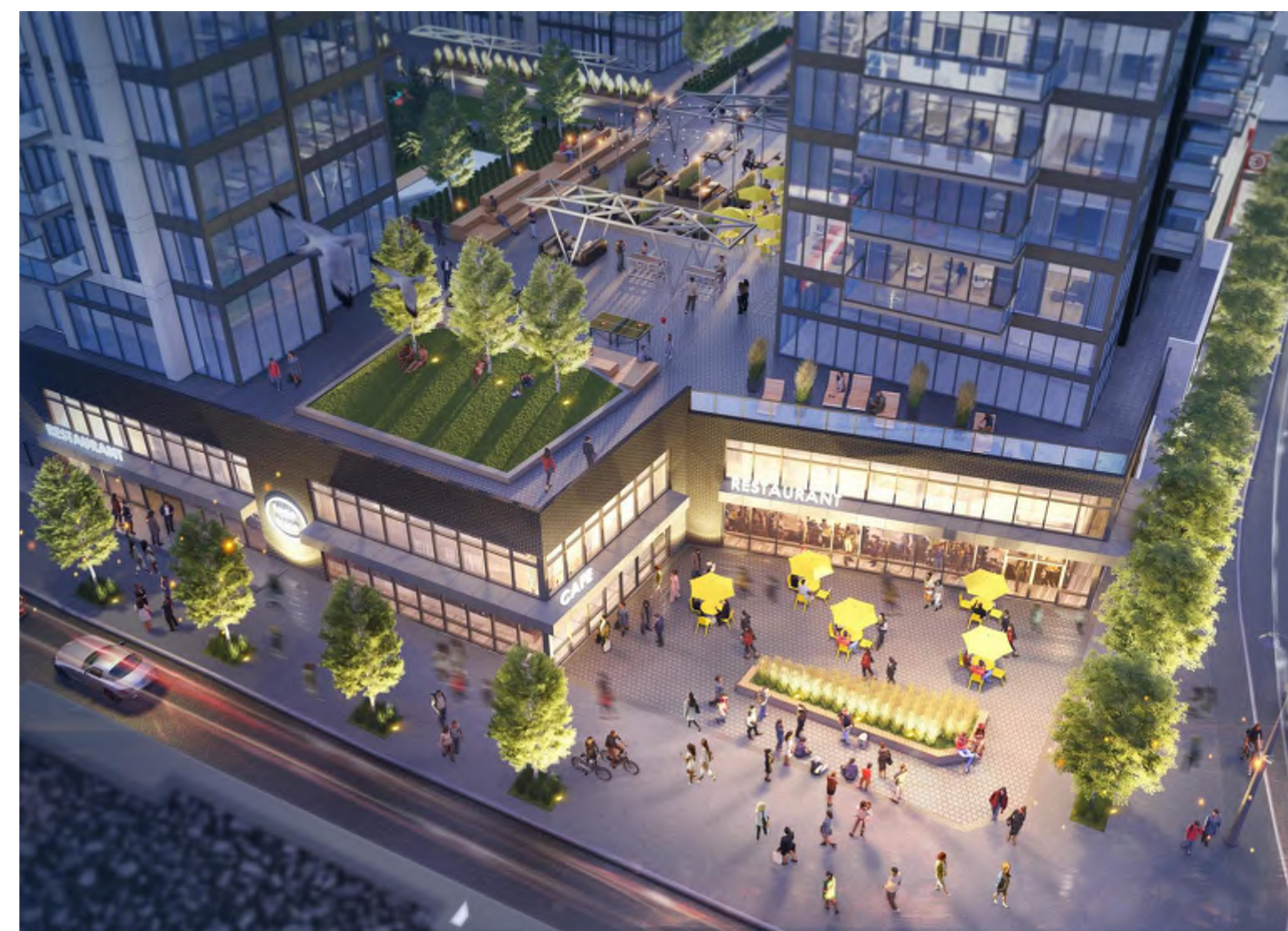
④ NORTH EAST CORNER
