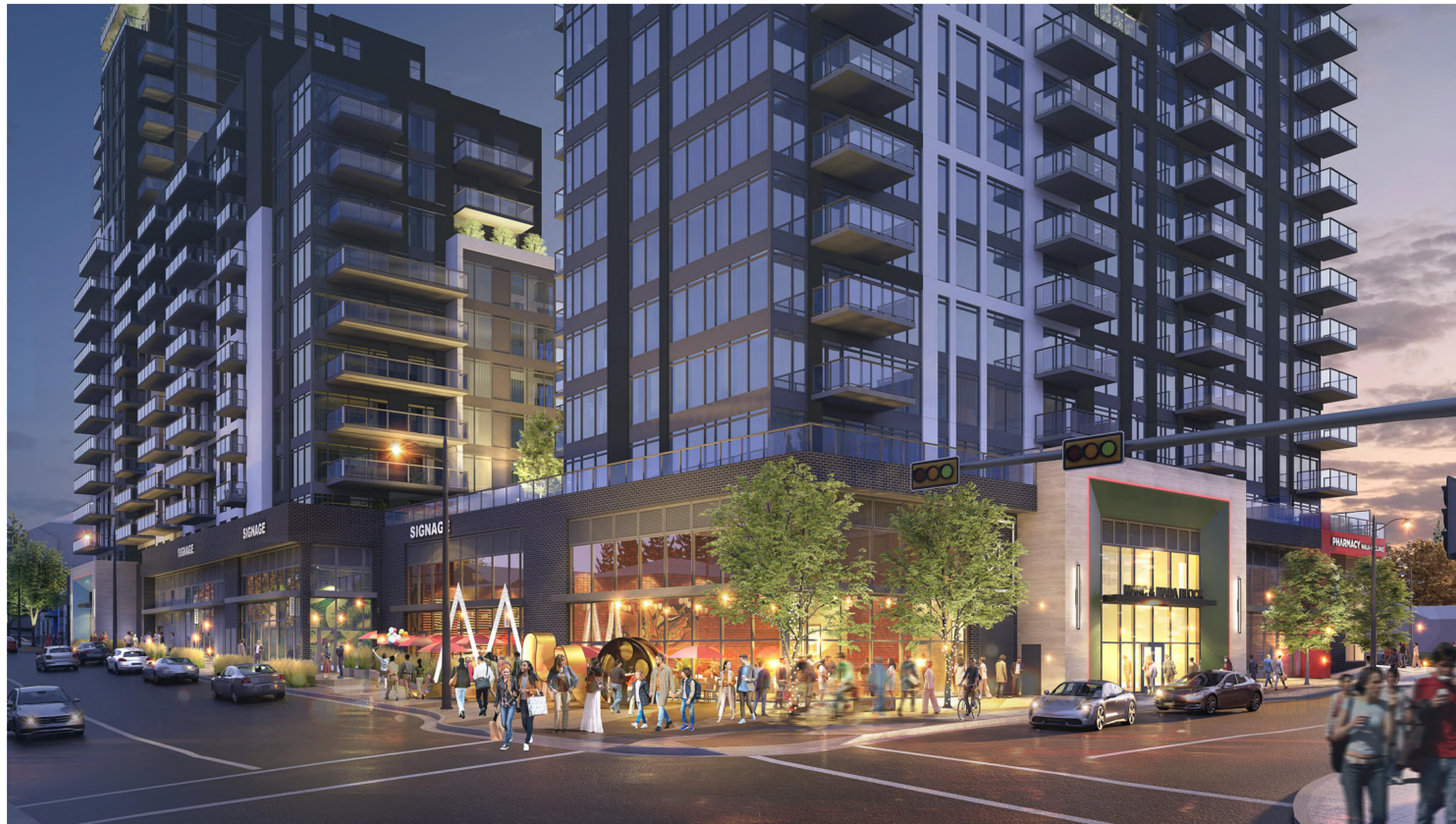
① SOUTH EAST CORNER
