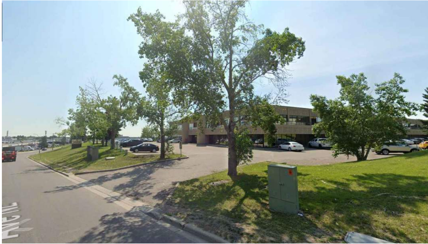
PHOTO 3: Site from NW, north vehicle access
