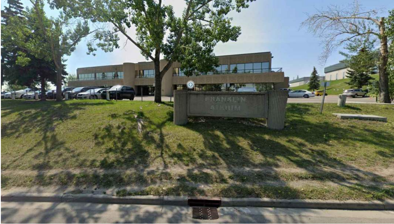
PHOTO 6: North building monument sign (typical at south)
