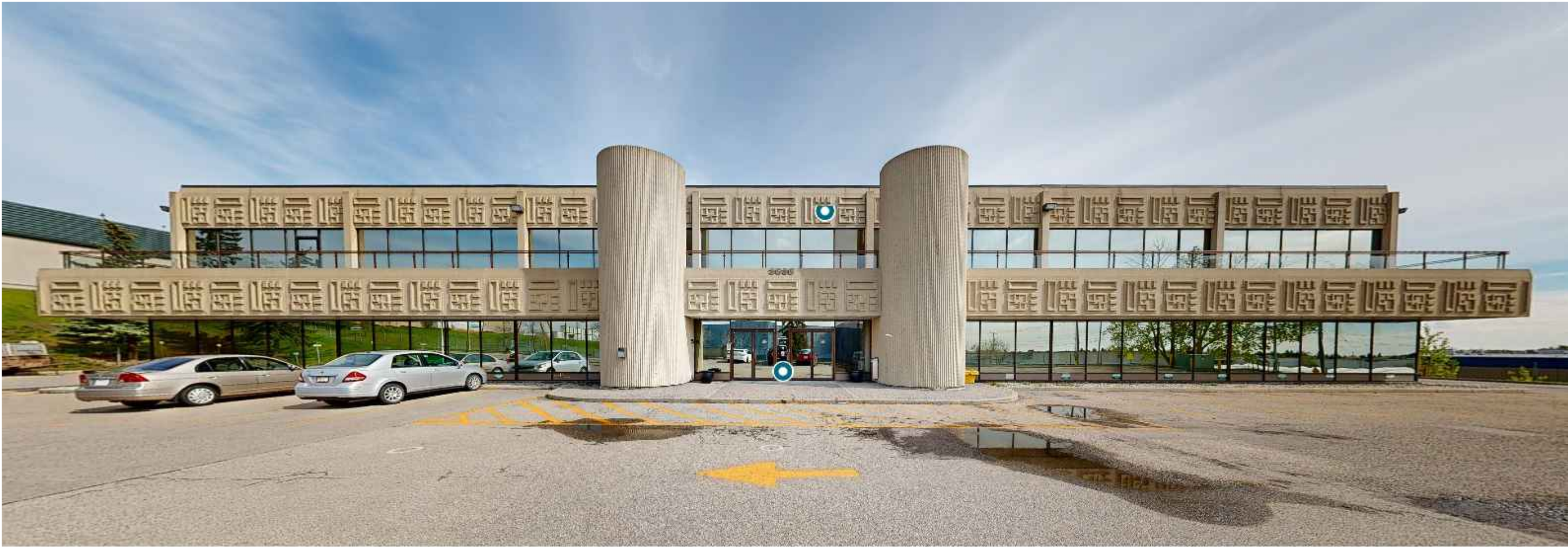
PHOTO 1: South building elevation and entrance (typical at north)
