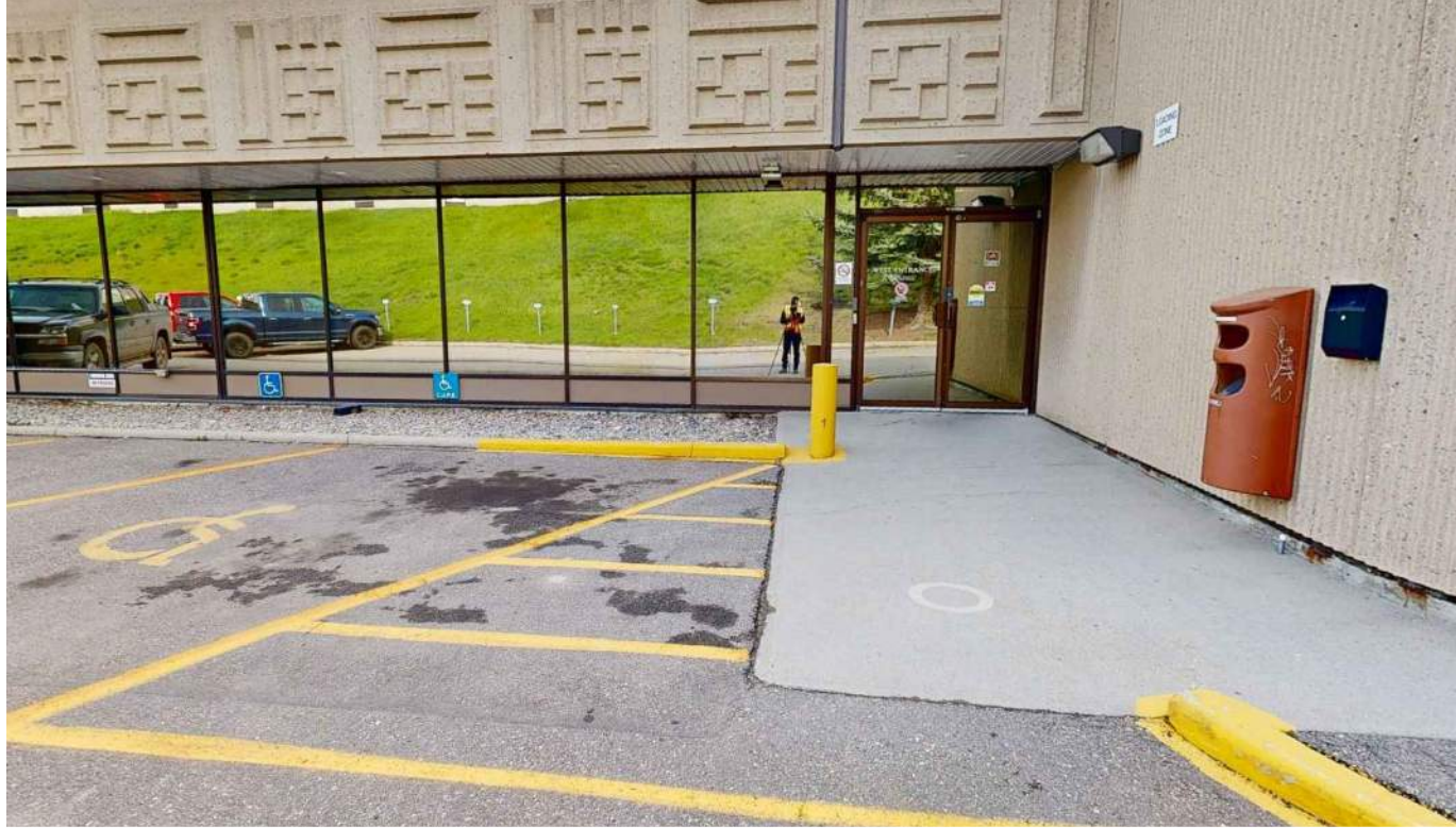
PHOTO 7: Principal entrance (fire department access)
