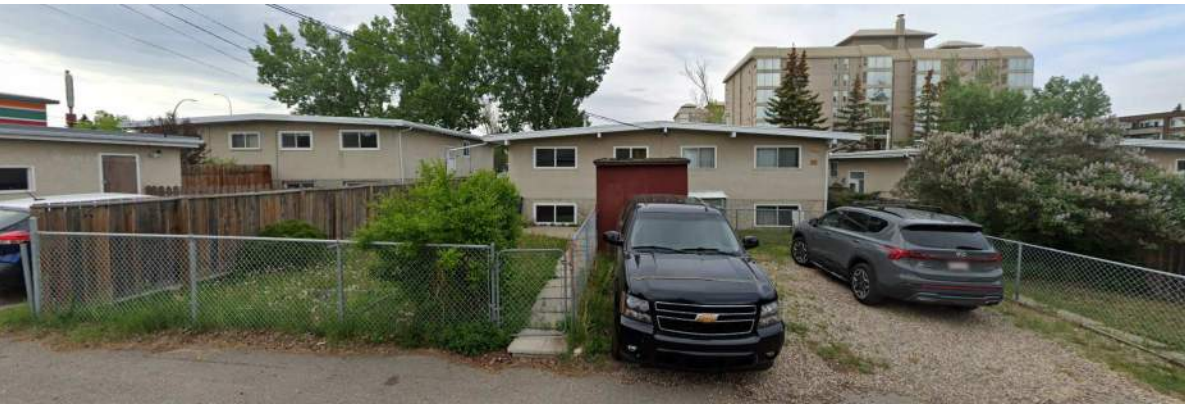
VIEW 2 - SOUTH (REAR)
