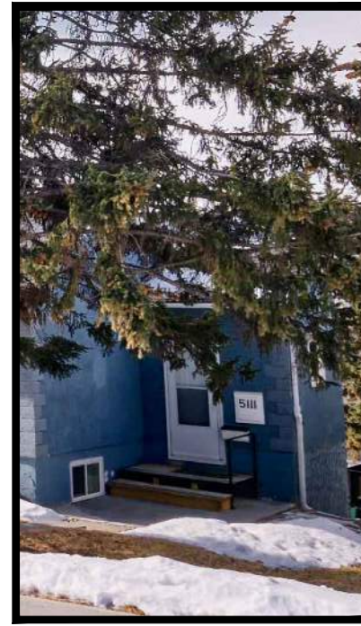
NORTHWEST "RIGHT ELEVATION" VIEW NORTHWEST OF PROPERTY LOOKING SOUTH
