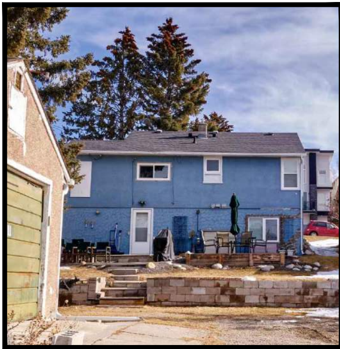
SOUTH "REAR ELEVATION" VIEW SOUTH OF REAR YARD LOOKING NORTH
