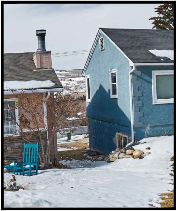
EAST "LEFT SIDE YARD" VIEW NORTHEAST CORNER OF PROPERTY LOOKING SOUTH
