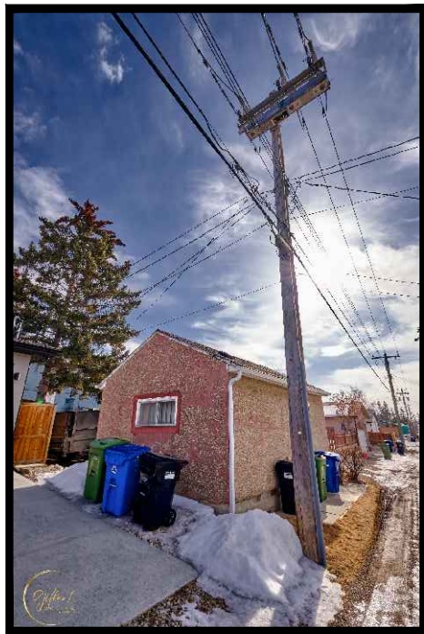
SOUTHWEST "LANE" VIEW NORTHWEST CORNER OF LANE LOOKING EAST
